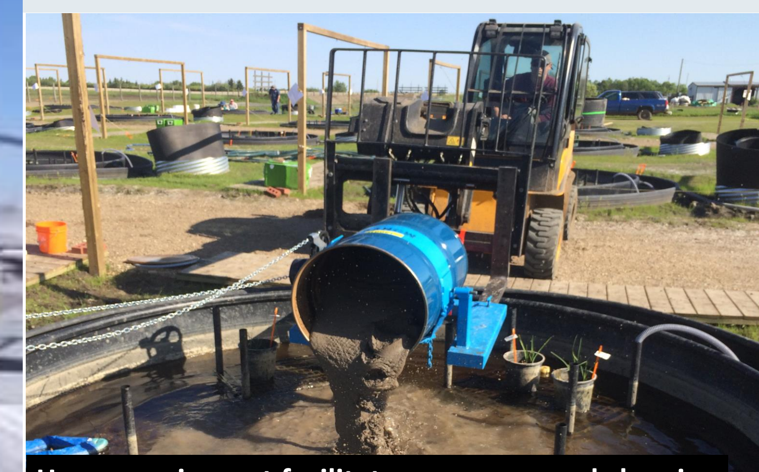
Heavy equipment facilitates exposure and cleaning
